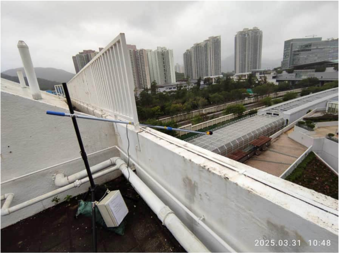
Overview of monitoring station NM2
