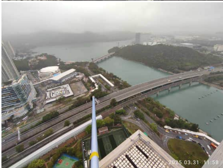
Overview of monitoring station NM1
